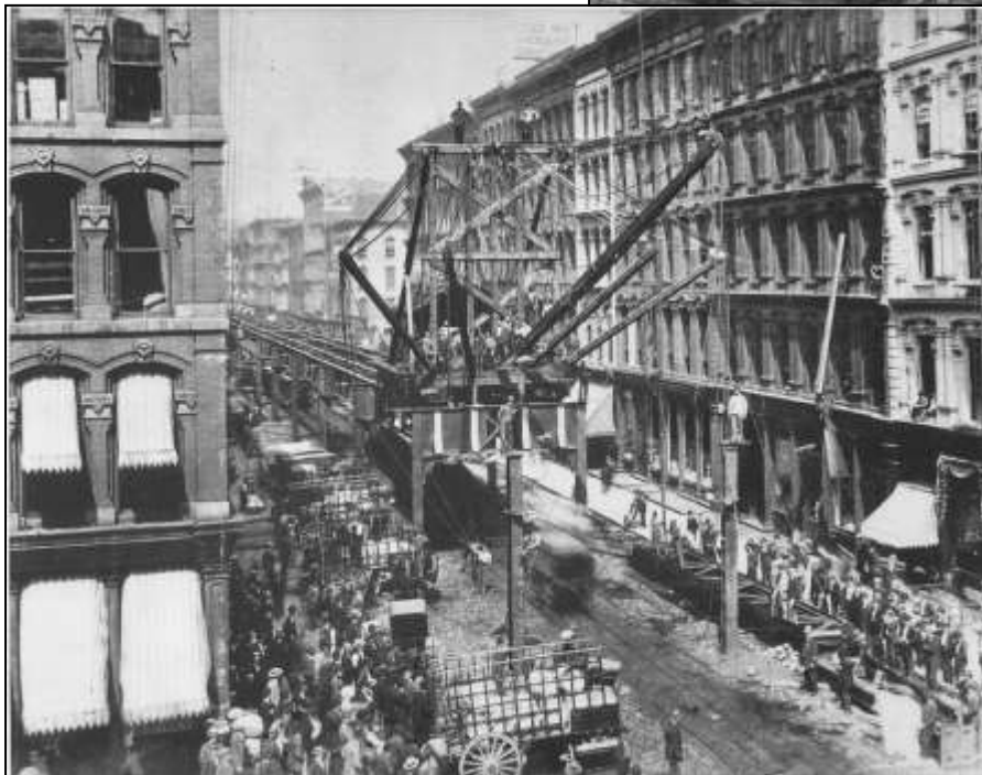
Construction of Chicago's transit system in 1895
