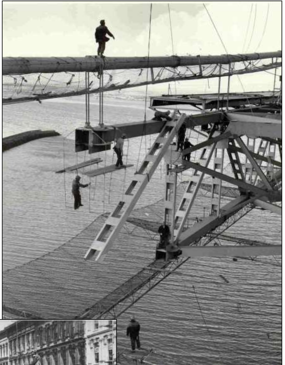
Construction begins on the Forth Road Bridge in November 1958
